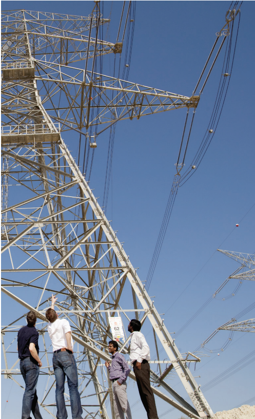
400 kV tension tower: 2 systems for a quadruple bundle
